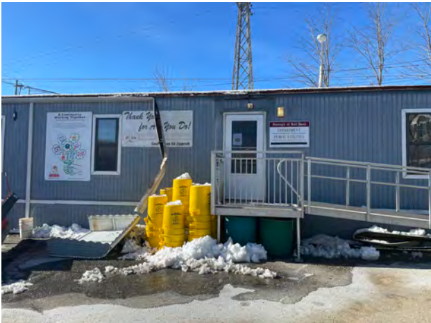
DPW main office
