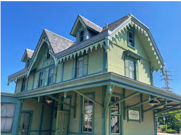
Lot 41-3, historic train station building
