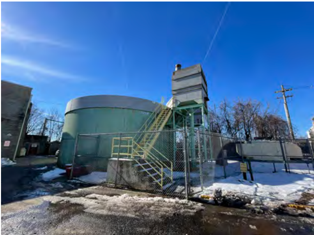
Water treatment tank
