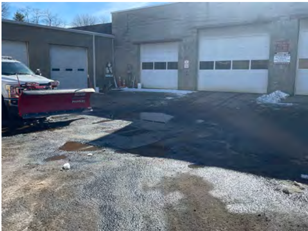
DPW garage bays
