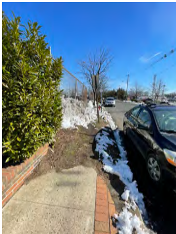
Missing sidewalk on Herbert Street
