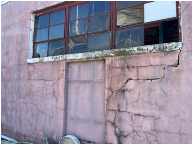
DPW storage building
